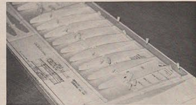
Wings are constructed rather conventionally. Airfoil is slightly curved on the bottom, so shims are needed at LE and TE for flat surface.
